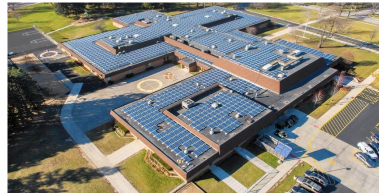
Solar panels installed at Butterfield Elementary (C & E Solutions, Handout)
